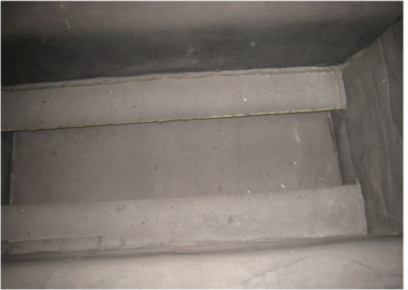
The shaft - seen from above.
